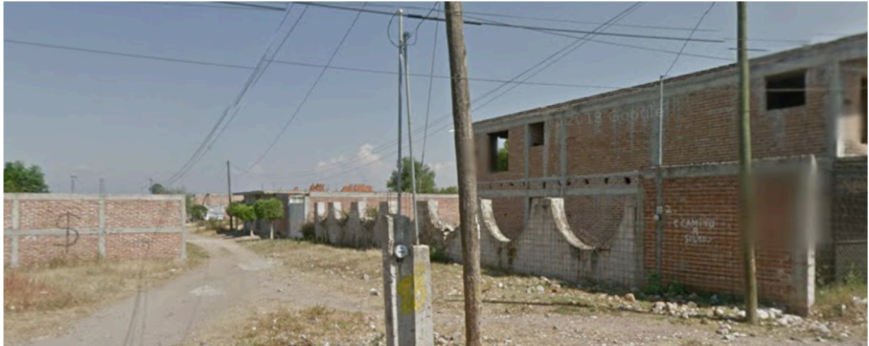
Fig. 4: The same building in Fig. 3, visible on Street View at the intersection of Felipe Angeles and Galeana.
