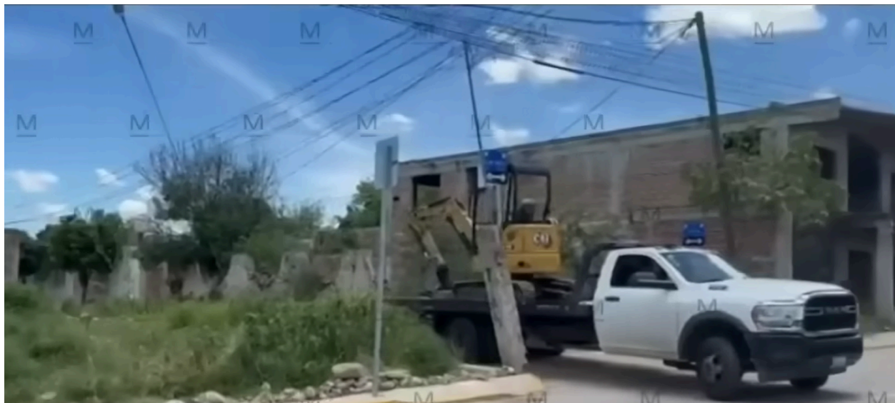
Fig. 3: An image of an excavator arriving at the site (at the intersection of Galeana and Felipe Angeles), which is off-camera to the left
